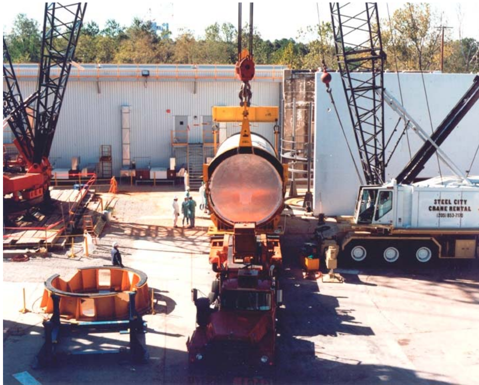
Figure 13. A variety of cranes will be used to move IVGVT hardware from transportation facilities to Test Stand 4550.
