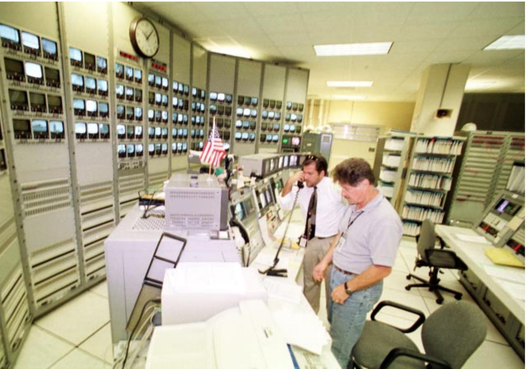
OTV lead technician, and Chris Perri, NASA OTV systems engineer, observe several camera views of processing areas in OTV Master Control in the Launch Control Room. The video wall (left) is used to monitor all KSC OTV camera locations.
